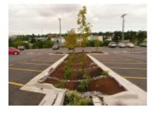
(d) A parking lot with permeable concrete floor and bio-swale for stormwater collection (Source: flickr.com)
