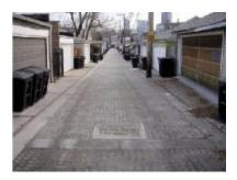
(a) Alley renovated with permeable paving located in Chicago, Illinois (Source: US EPA - Document No. EPA-833-F-08-009)
